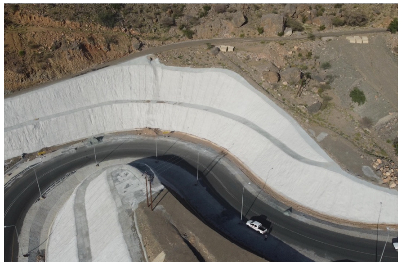
Aerial view of completed ConstruckSlope Plus
